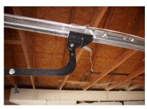
The small overhead door springs are weak or out of adjustment, and should be serviced by a qualified overhead door contractor. (Door does not stay up by itself when lifted)
