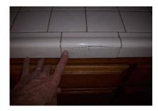
An open seam between the sink and the counter top needs to be caulked or re-caulked to forestall moisture intrusion.
